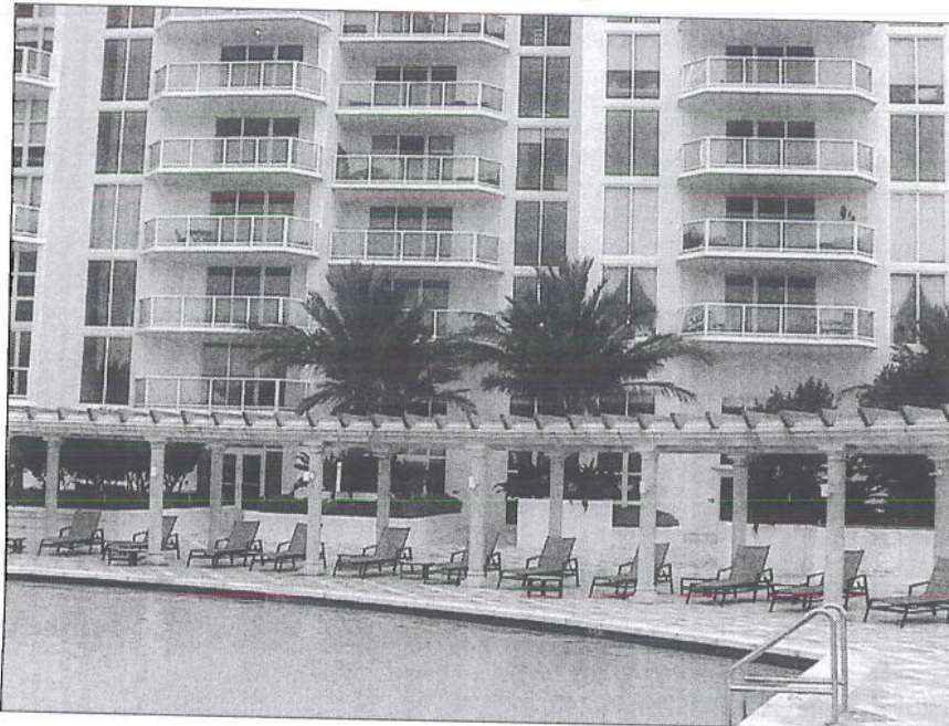
The Peninsula II condominium in Aventura has had problems with defective Chinese drywall. FILE PHOTO
